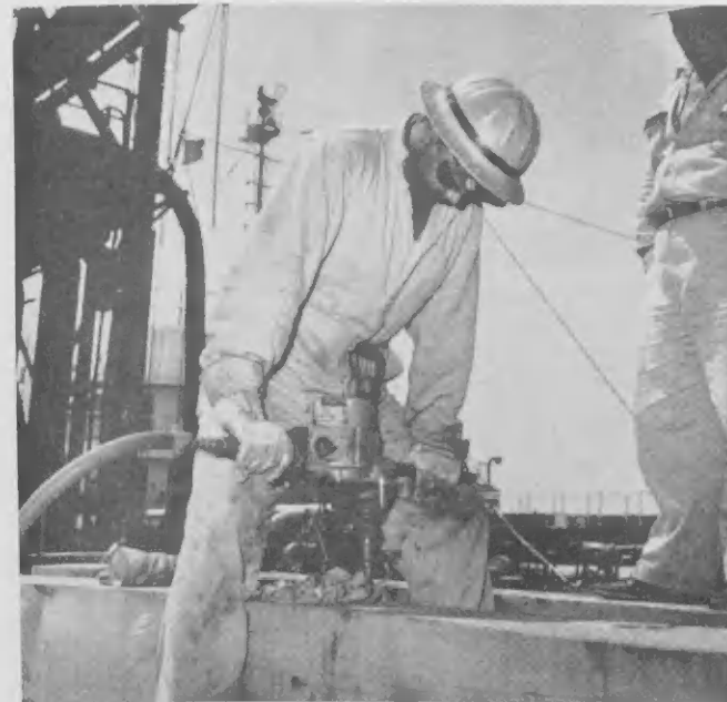
DOWELS FORMED in greenhart are turned in the Carpenter Shop and then driven into openings in the timbers where bolts had been driven through. Glued and sawed flush, the result is a closed, smooth finish on the timber's outboard side. This was done 4000 times along the length of the pier.
